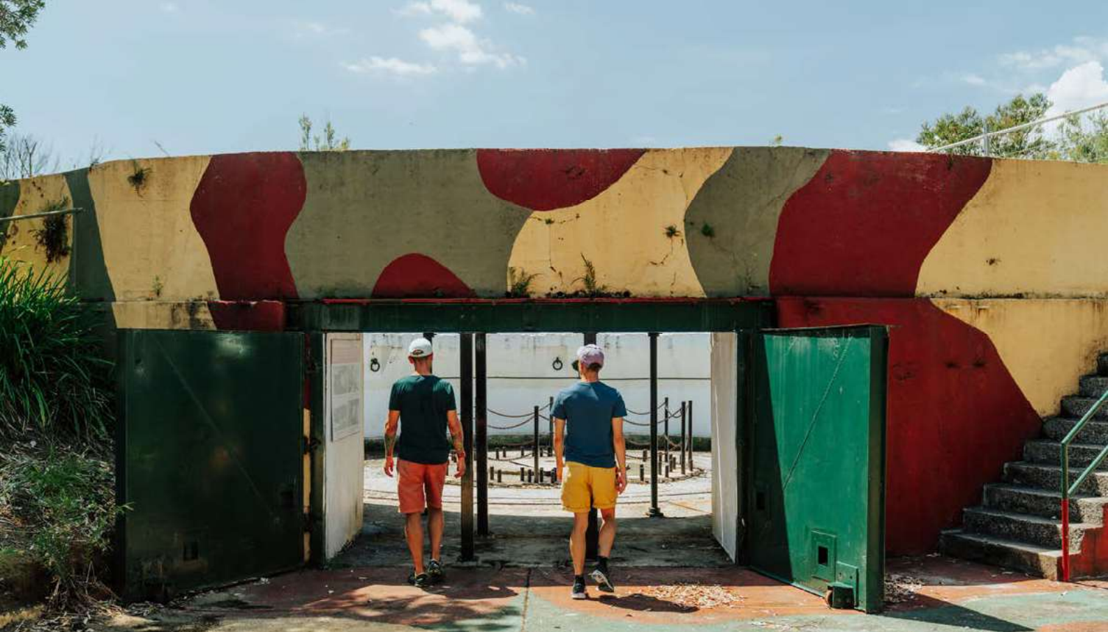
Image: The No 2 Gun Emplacements located at North Fort, North Head Sanctuary
