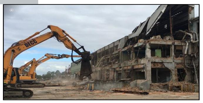
Figure 5 – Process of Steelwork with Shear Attachment
