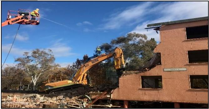
Figure 3 – Demolition of Structures with Large Excavators and Rubble Mound
