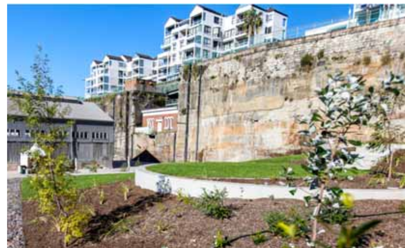
Figure 46: View of the upper level and Exhauster House
