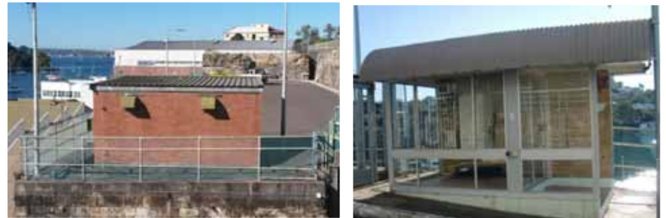
Figure 24: POL Store and Car Park Guardhouse
