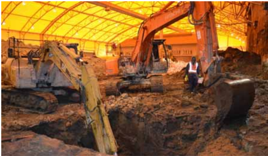
Figure 10: Excavated Tar Pit, Retort Building in the background (2013)
