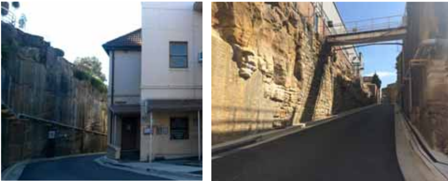
Figure 27: Access Road and Pedestrian Bridge
