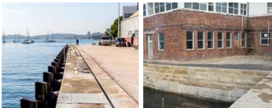
Figure 21: Submarine Wharf and Seawall
