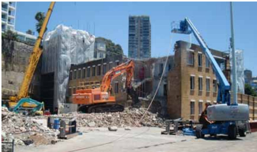
Figure 9: Demolition of Naval Administration Building (2010)
