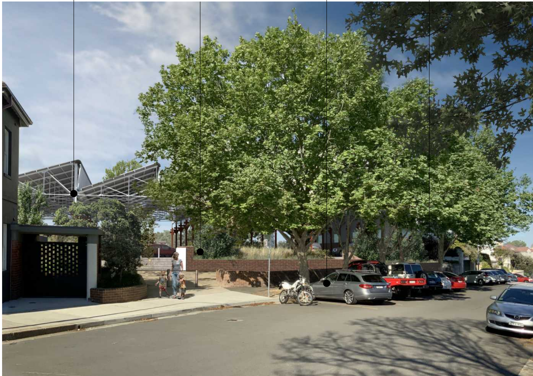
Fig.45 RANTME Factory and Entry Forecourt
