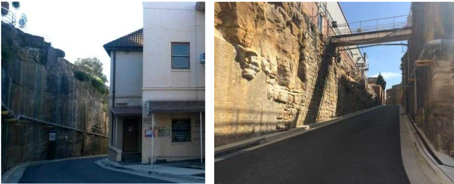
Figure 27: Access Road and Pedestrian Bridge
