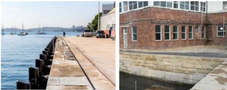
Figure 21: Submarine Wharf and Seawall
