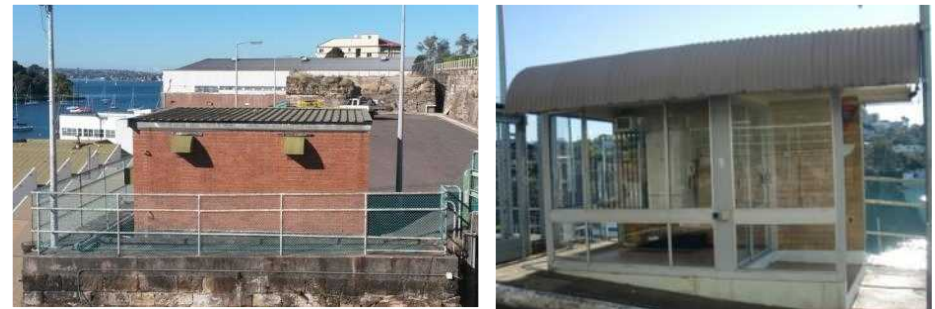
Figure 24: POL Store and Car Park Guardhouse
