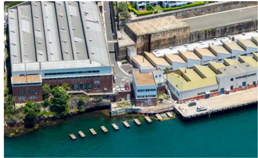
Figure 12: Retained Wharf Headstocks
