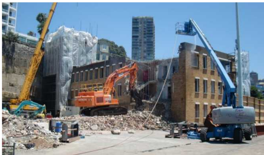
Figure 9: Demolition of Naval Administration Building (2010)
