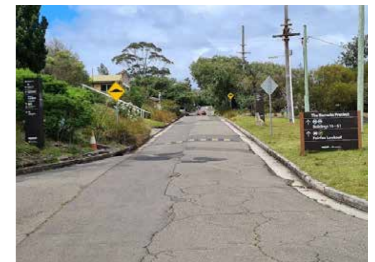
Figure 122. North Fort Precinct Road in the Barracks Precinct
