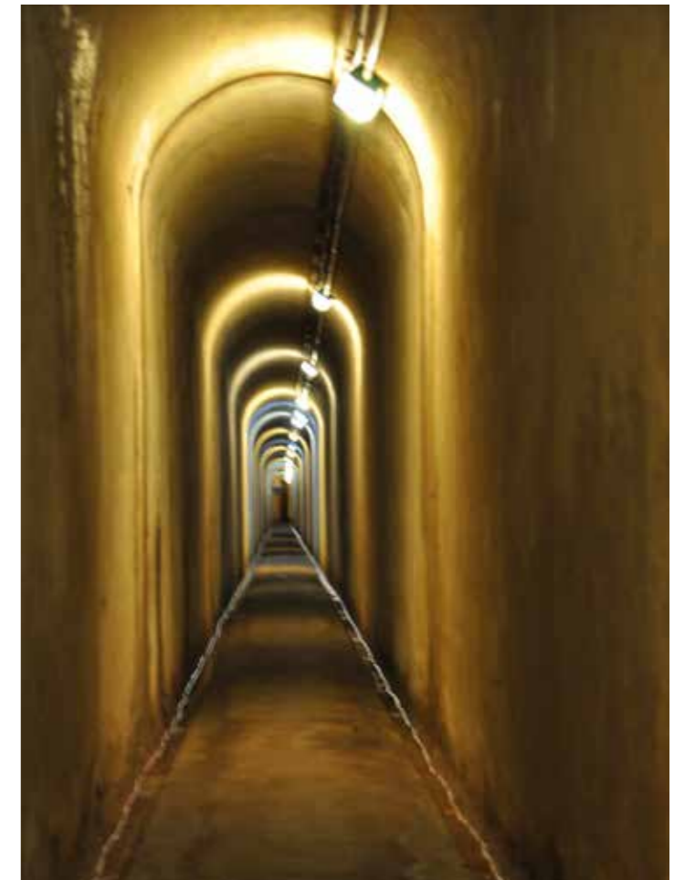
Figure 38. Tunnels at North Fort. Source: Harbour Trust
