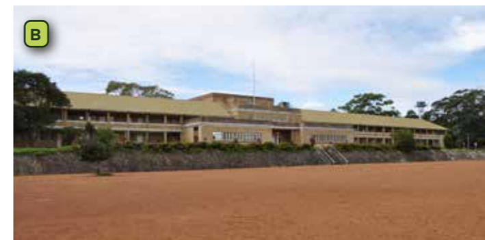
Figure 97. Main Barracks Building (B1)
