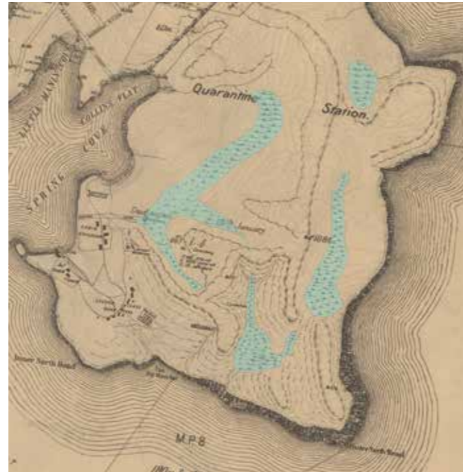
Figure 80. Hanging Swamp throughout the North Head
