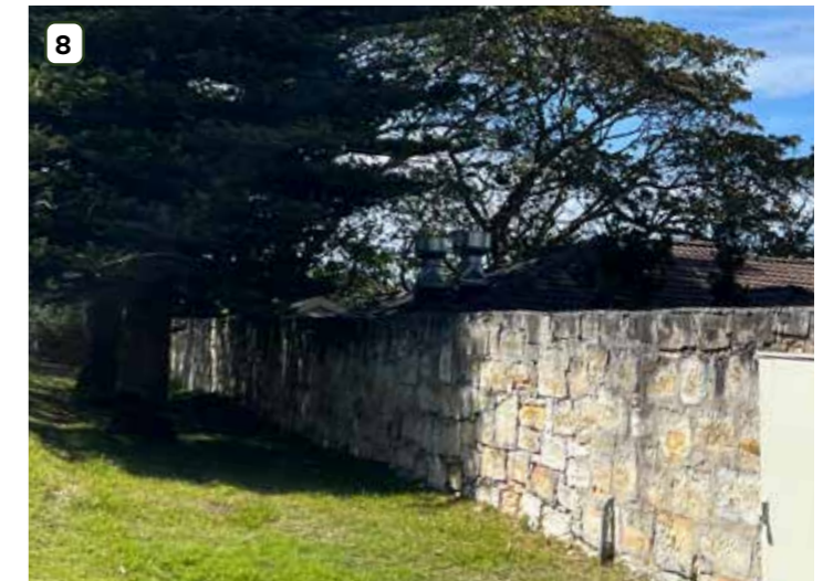
Figure 115. North Fort Precinct sandstone perimeter wall
