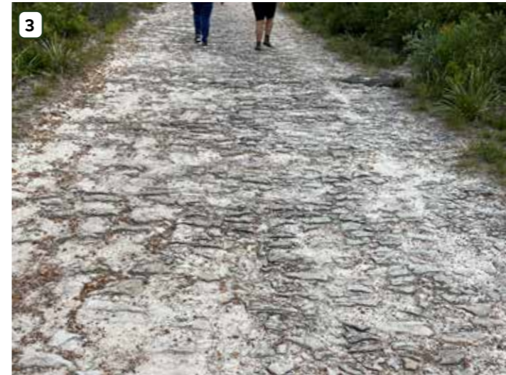
Figure 107. Current cobblestone construction
