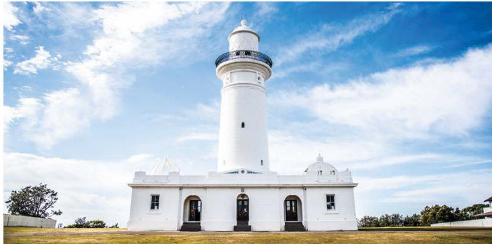
Macquarie Lightstation, Vaucluse.
